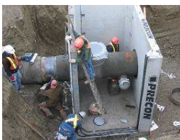
Municipal Water Feeder Main Extension
