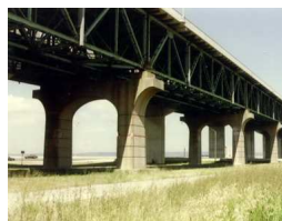
Aesthetic Guidelines for Bridges
