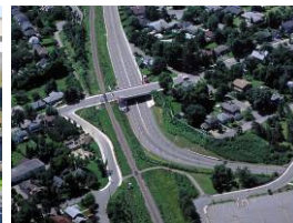
Southeast Transitway Stage II
