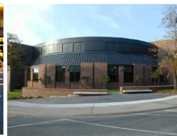
Transit Control Centre
