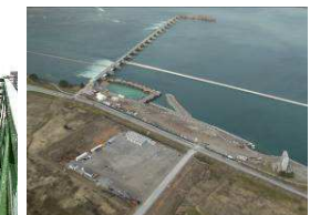
Niagara Tunnel Intake Works
