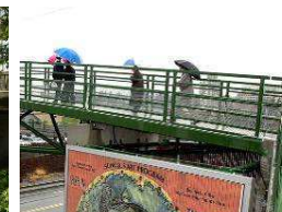
Pedestrian Bicycle Overpass
