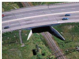
Road Railway Overpass
