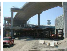
Access Road and Runway Lighting Upgrade
