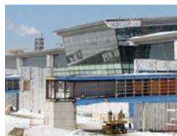
New Terminal Construction
