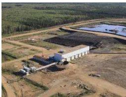
Telecommunications Infrastructure for Industrial Site
