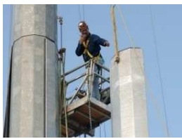
Turnkey Tower Reinforcement
