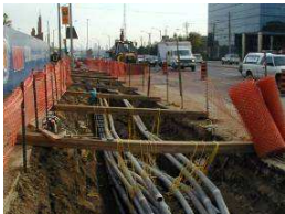
New Outside Plant Infrastructure
