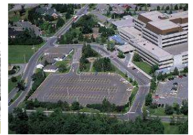
Civil Works Projects for Health Sciences Center
