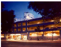
New Parking Garage and University Bookstore Complex
