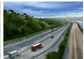
South Fraser Perimeter Road Design-Build
