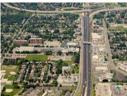
Reconstruction and Widening of Highway
