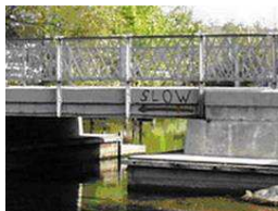
Bridge Rehabilitation and Reconstruction
