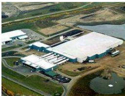
Regional Co-Composting Facility
