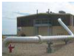
Underground Pipe Fire Protection System Upgrades
