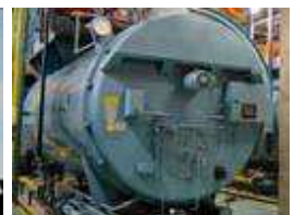
Boiler Demolition and Replacement
