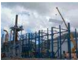
Power Station Redevelopment
