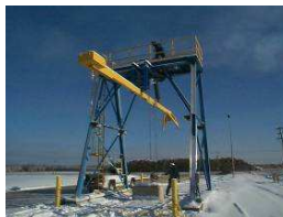
Veneer Plant Site Improvements
