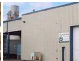
Plywood Plant Firewater Pump Station
