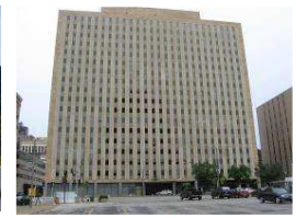
Assessment of Data Center
