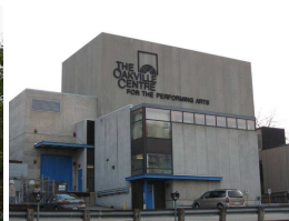
Municipal Building Condition Assessments
