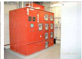
Municipal Government, Emergency Medical Services (EMS) – Critical Infrastructure Upgrade
