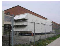
Provincial Government – Standby Diesel Generator Installation for Data Centre
