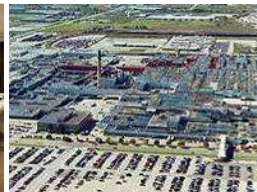
Ontario Fire Code Part 4 Audit, Flammable and Combustible Liquids
