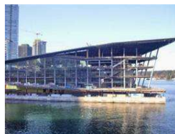
Convention Center Expansion Project
