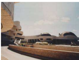
Museum Building Envelope Review
