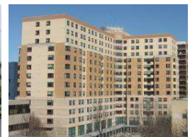
Exterior Wall Repairs for University Residence
