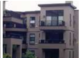
Building Envelope Rehabilitation for Three Storey Wood Framed Structure
