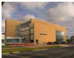
Campus Research Facility
