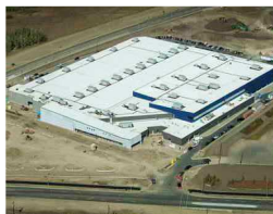
South Edmonton Transit Facility
