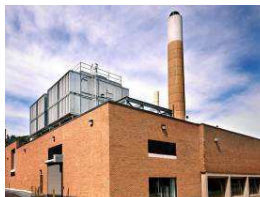
Central Utility Plant & Cooling Tower Upgrade Project
