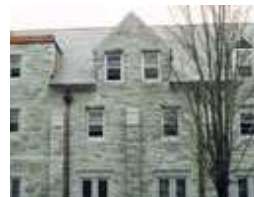
Technical Audits Envelope Rehabilitation
