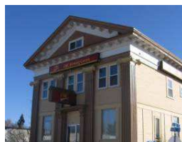
CIBC Building Envelope Condition Assessment
